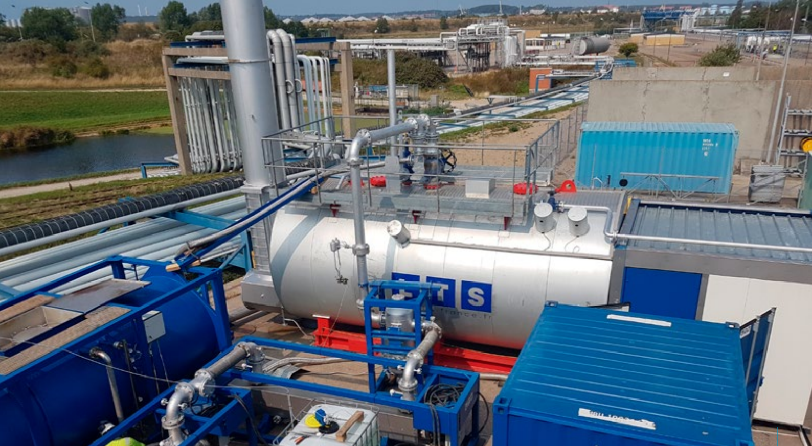
Temporary installation to bridge routine boiler maintenance at Equinor Refinery Denmark A/S. 16 000 kg/h Steam Boiler with super-heated water boiler to bring up the temperature to +225C° at 18 bar.
