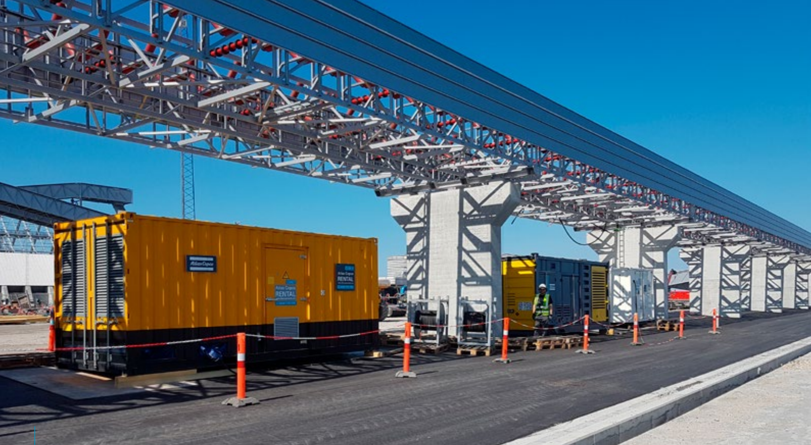
Temporary back-up solution for HOFOR in Denmark: a fuel efficient 1250-kVA diesel generator (400V) connected with a 2500-kVA transformer that converts and supplies cranes with 10 kV voltage.
