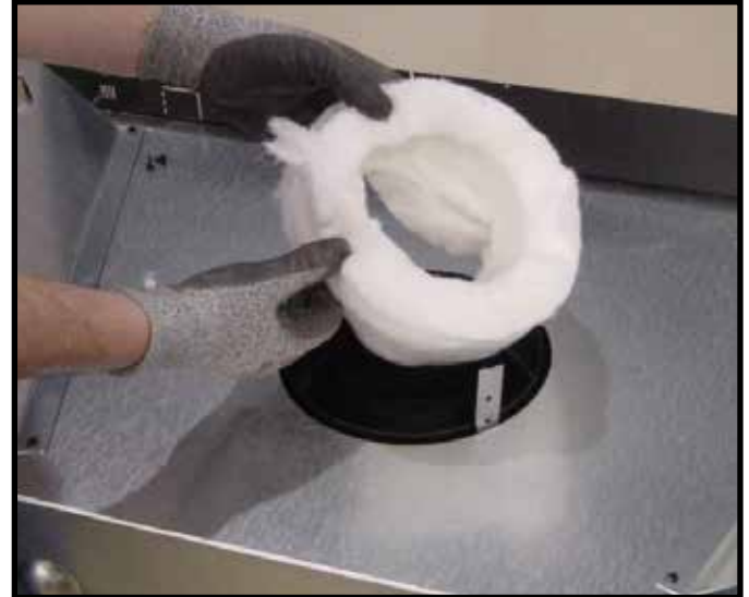
Figure 6.5 (Generic Fireplace Shown) Remove the insulation from the outer vent pipe. For rear venting there is no insulation in the outer vent pipe.
