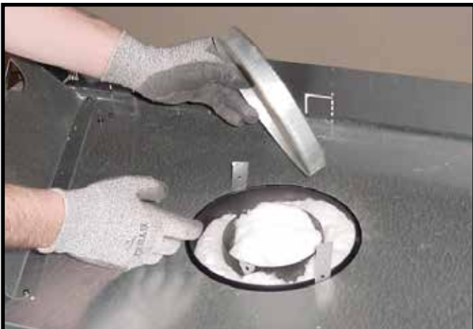
Figure 6.3 (Generic Fireplace Shown) Remove the seal cap.
