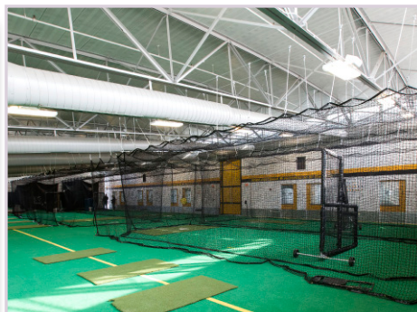
Jacobson Hitting Facility
