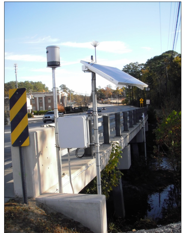
The GIL-A Monitoring Station
