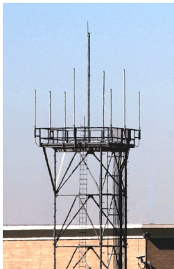
This is one of six communications towers at NCT. The center pole is probably for lightning protection. The antennas may be something on the order of: www.wade-antenna.com/TACO/FAAApproved.pdf
