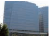
Guangzhou FA Center MITSUBISHI ELECTRIC AUTOMATION (CHINA)LTD.
