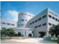
Taichung FA Center MITSUBISHI ELECTRIC TAIWAN CO.,LTD
