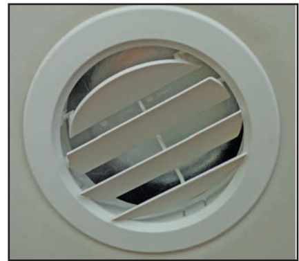
Figure 3-4: Round air vent
