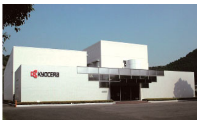
Kyocera Kagoshima Training Center
