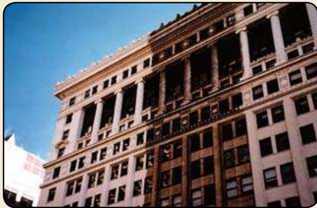
Insurance Exchange, Chicago, Ill.—exterior cleaning with PROSOCO products.
