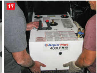
(14) Brass tube is inserted into the end of the PEX tubing to provide rigidity for the clamps. (15) The PEX tubing is connected to the heat exchanger's rubber hose using a very strong clamp installed by a tool designed for this purpose. (16) Very specific instructions are provided for positioning the mounting plate that secures the boiler housing. (17) Boiler housing is heavy, so two installers carefully position it into a compartment in the front portion of the fifth-wheel.
