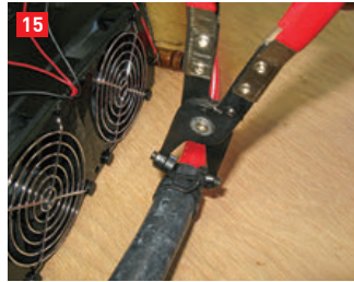
(14) Brass tube is inserted into the end of the PEX tubing to provide rigidity for the clamps. (15) The PEX tubing is connected to the heat exchanger's rubber hose using a very strong clamp installed by a tool designed for this purpose. (16) Very specific instructions are provided for positioning the mounting plate that secures the boiler housing. (17) Boiler housing is heavy, so two installers carefully position it into a compartment in the front portion of the fifth-wheel.
