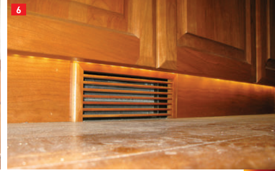
(4) Boiler tank is fitted in a prepared cabinet. Control panel is mounted above the main box. It provides all the diagnostic information for smoothing operation. (5) Access to this heat exchanger is through the floor of a cabinet structure. (6) Nice-looking heat exchanger grilles are used to blend in with cabinetry.
