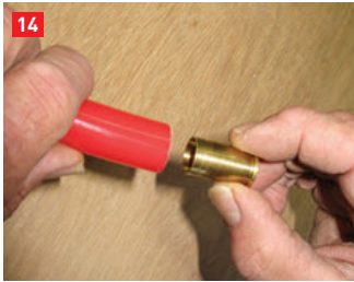
(14) Brass tube is inserted into the end of the PEX tubing to provide rigidity for the clamps. (15) The PEX tubing is connected to the heat exchanger's rubber hose using a very strong clamp installed by a tool designed for this purpose. (16) Very specific instructions are provided for positioning the mounting plate that secures the boiler housing. (17) Boiler housing is heavy, so two installers carefully position it into a compartment in the front portion of the fifth-wheel.
