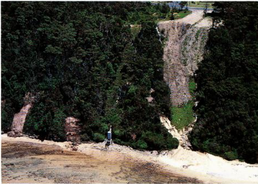
Figure C7.2 Landslip Failure of Coastal Bluff, Bateau Bay, Wyong Shire
