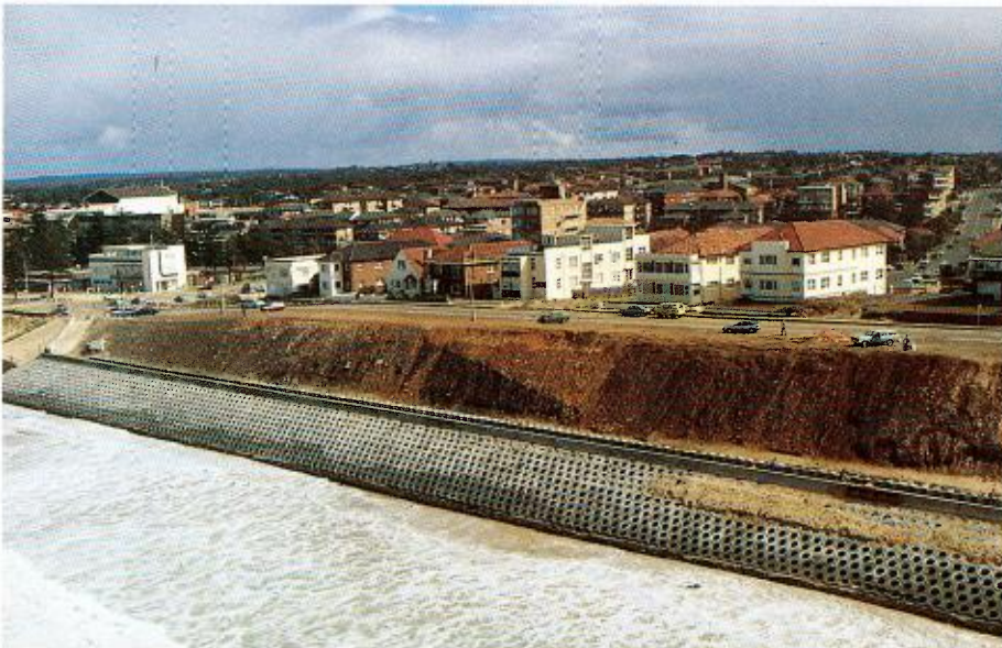
Figure D6.1(d) Semi-rigid Seawall of SEABEES®
