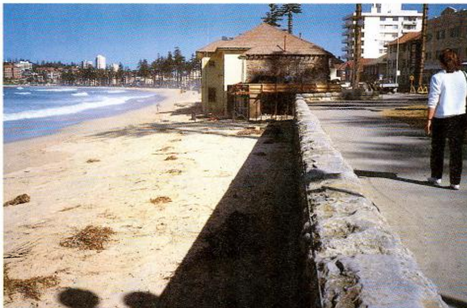
Figure D6.1(a) Rigid Vertical Seawall
