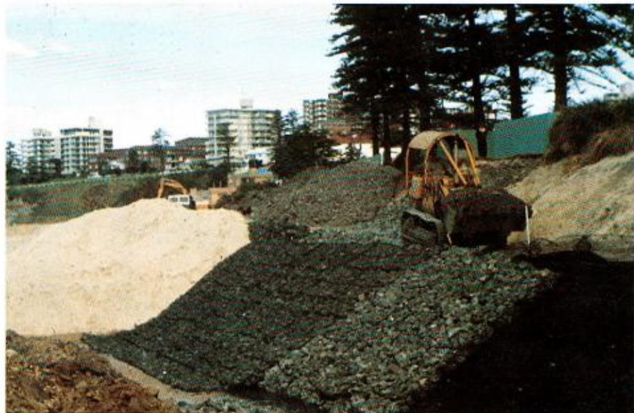
Figure D6.1(c) Sloping Gabion Seawall
