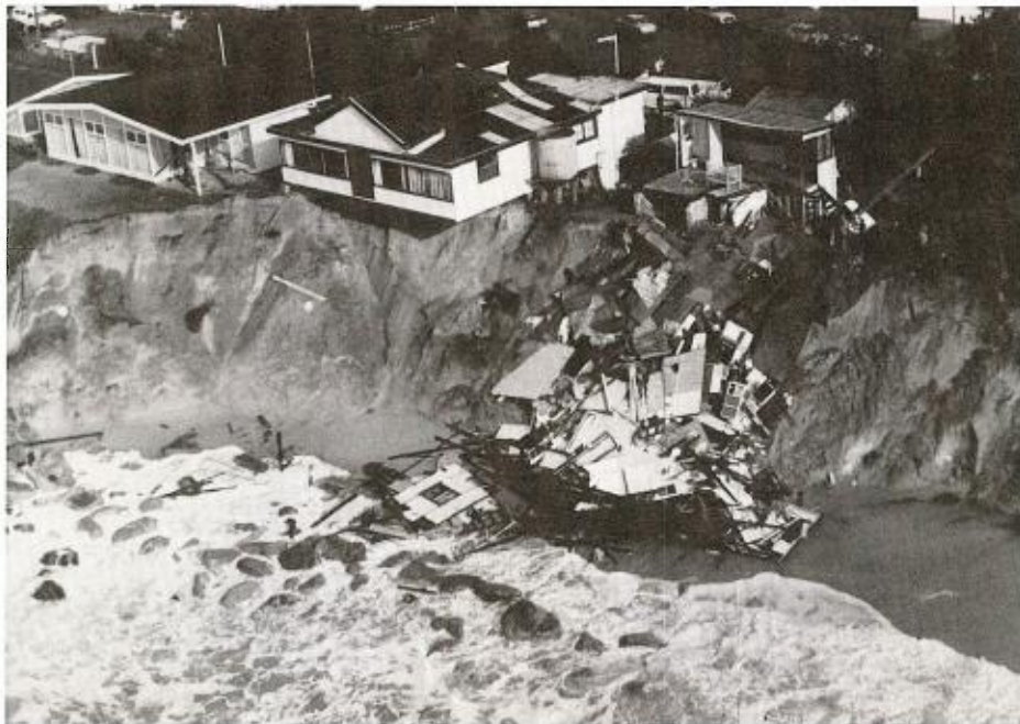
Figure C2.1 Undermining and Collapse of Buildings Caused by Beach Erosion
