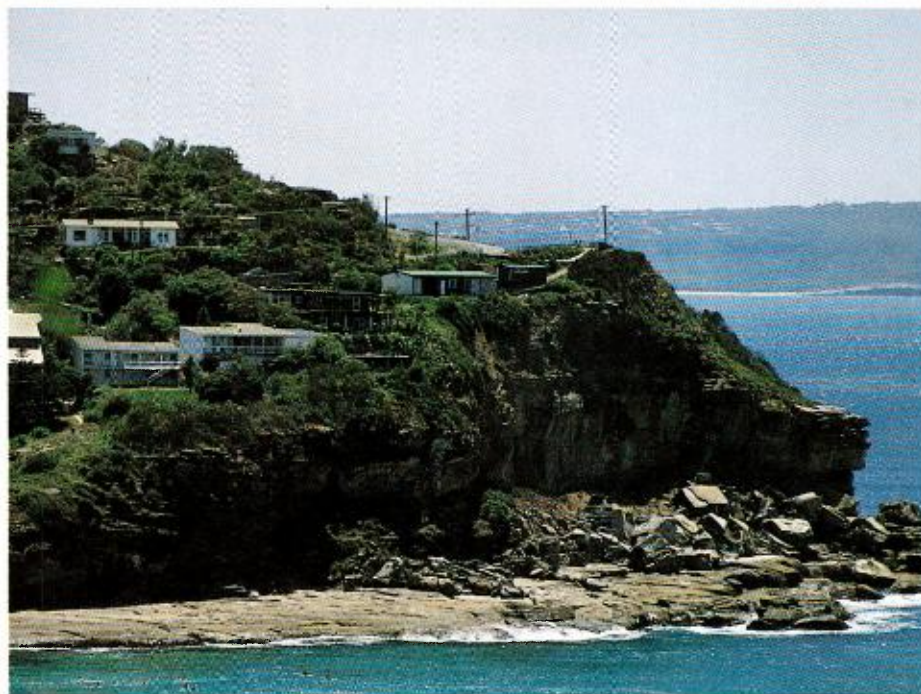
Figure C7.3 Cliff Collapse, Whale Beach, Warringah Shire
