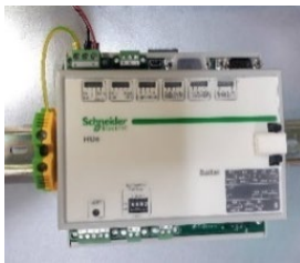
Figure 4 – Example of earthing for EMC.
