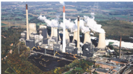
Figure 5.4 – ABB AG Power Technology Systems, 2006
