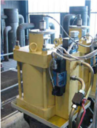
Figure 5.8 – Upgraded turbine valve servo drive photo, (ABB Utilities GmbH, 2004)
