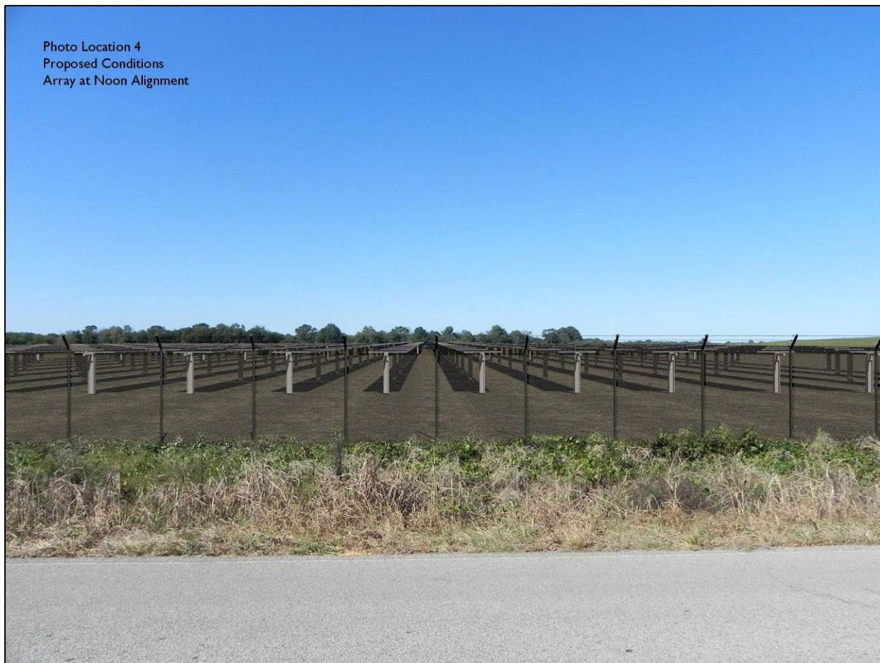
Photo 3.5-19: A rendering of the Project with the panels in the position they would be at noon and during high wind events, horizontal.
