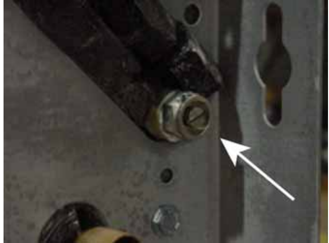
Figure 33. Manual coil air vent with Shrader fitting
