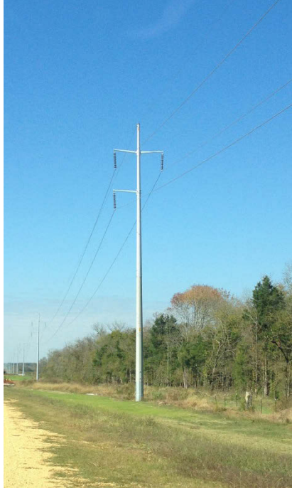
Figure 2-2. Typical Single Steel-Pole Structure
