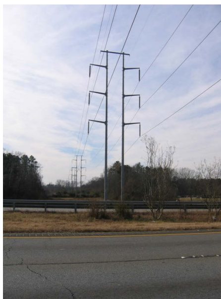
Figure 2-1. Typical Double Steel-Pole Structures, Double-Circuit Transmission Line
