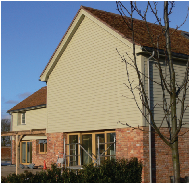
Post occupancy monitoring house in Berkshire
