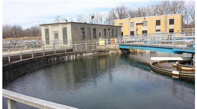
The City of Muncie Wastewater Treatment Plant
