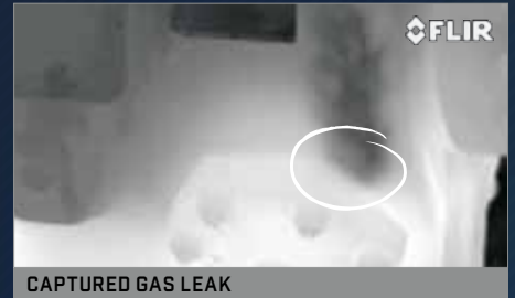
CAPTURED GAS LEAK
