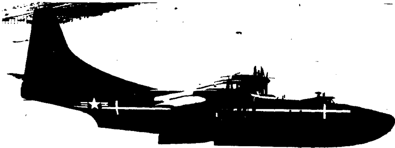
Powered by four Allison T-40 twin turboprop units, the 60-ton Convair XP5Y-1 was the world's first turboprop flying boat to fly.
