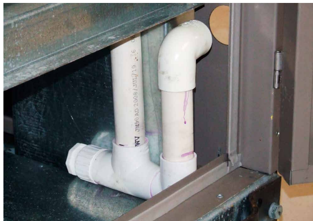
FIGURE 46 - CONDENSER TRAP
