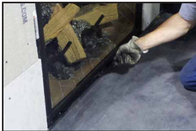
Figure 11.8. Securing Bottom Glass Clips
