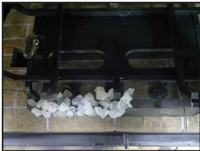
Figure 11.9. Install Teco-Sil
