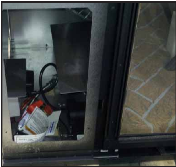
ACCESS THROUGH LEFT COLUMN (Prior to installation of non-combustible board)
