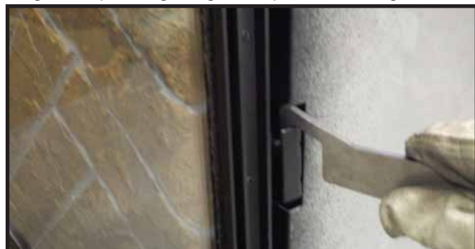
Figure 11.7. Securing Side Glass Clips
