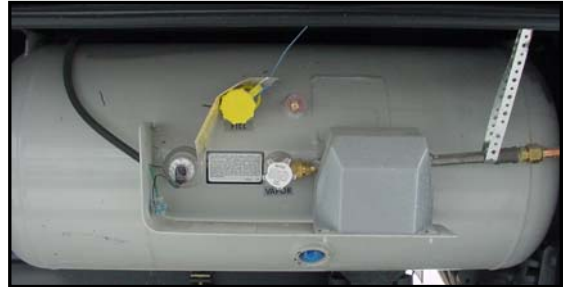
Figure 3-4. Liquid Propane Tank
