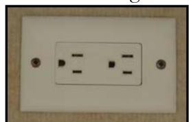
Figure 7-5. 120 VAC Receptacle
