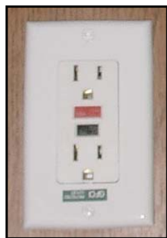
Figure 7-7. GFCI Receptacle
