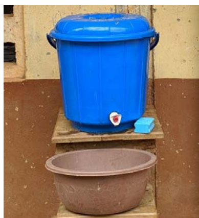
From left to right: Handwashing bucket with tap and basin to catch used water, Tippy tap, and Nudges, or visual cues, leading users to a handwashing station (Photo credits: Victoria Trinies, CDC)
