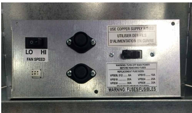
FIGURE 11 - UNIT SWITCH PLATE WITH ADA THERMOSTAT CONNECTION
