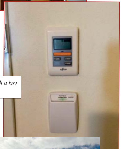
Slim Duct unit in soffit leading to the guest room.
