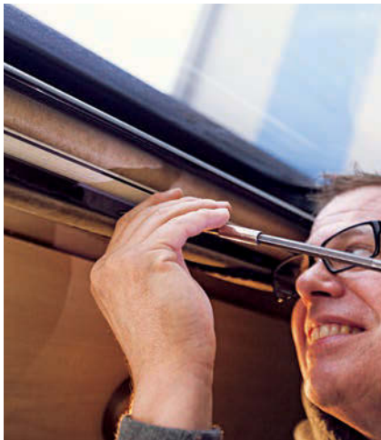
Auto-Motion shade is first installed in the valance on the bench and then attached to the wall as a package.
