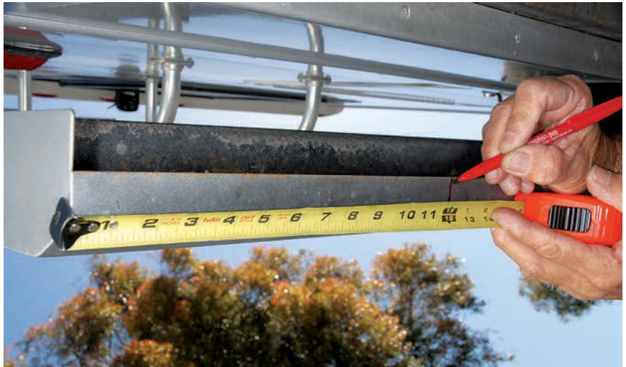
Measure carefully and mark the location for mounting each sensor bracket for proper operation of the SenseStat system.
