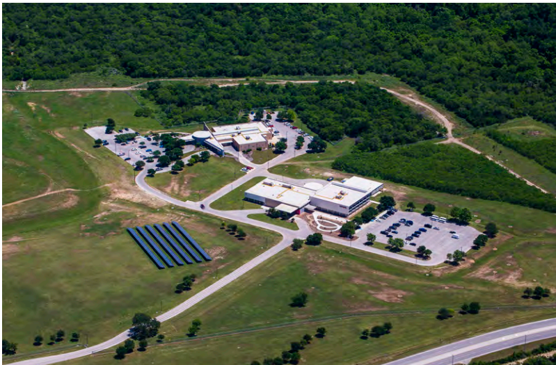
Toyota’s assembly plant in San Antonio, Texas, installed a 200-kilowatt ground-mount solar array to support the Visitor and Education Center and the Family Health Center.
