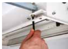
Single screw height adjustment
