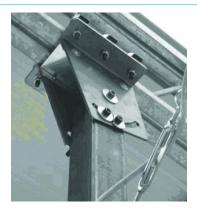
If the fan will be directly assembled to the metal structure of the building, it is necessary to use bolts M10 A2 screwed in the appropriate inserts, placed on the stand for the anchorage (two per side).
