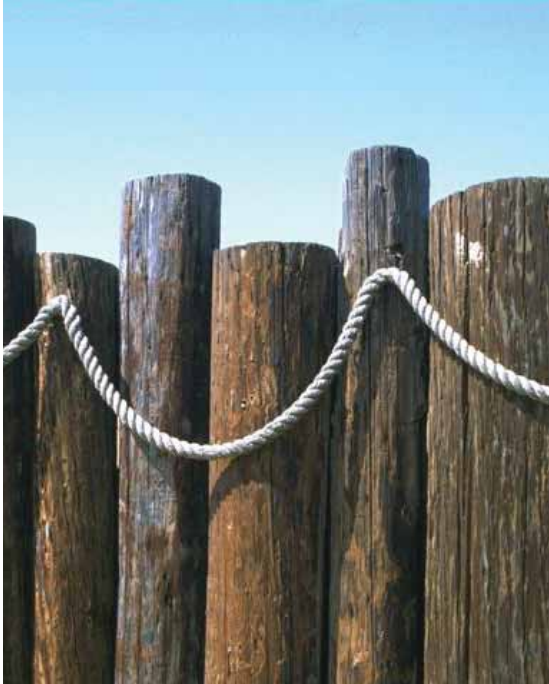
Figure 6. Wood used in docks and marine pilings should be treated to prevent damage by marine borers.
