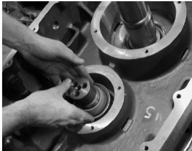
FIGURE 7-24 – OIL SEAL ON GATE ROTOR SHAFT ASSEMBLY
