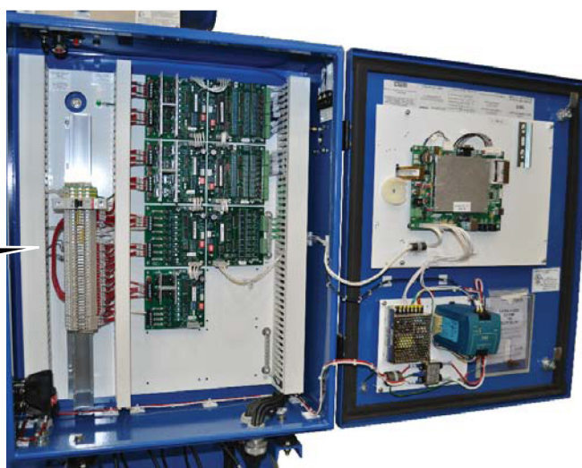
Figure 4-5. Wire Connections for Capacity and Volume Actuators
