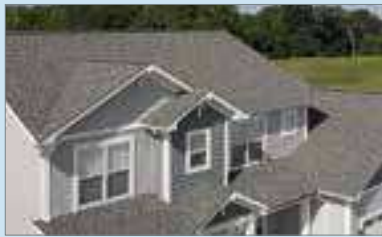
Roofing and Ventilation
