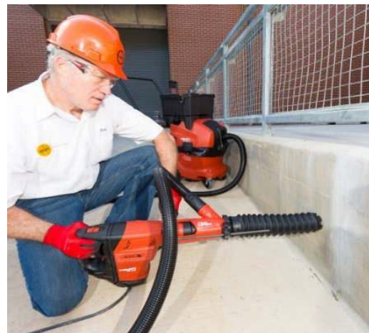
Worker drilling into concrete with a rotary hammer equipped with a shroud and dust collection system.
