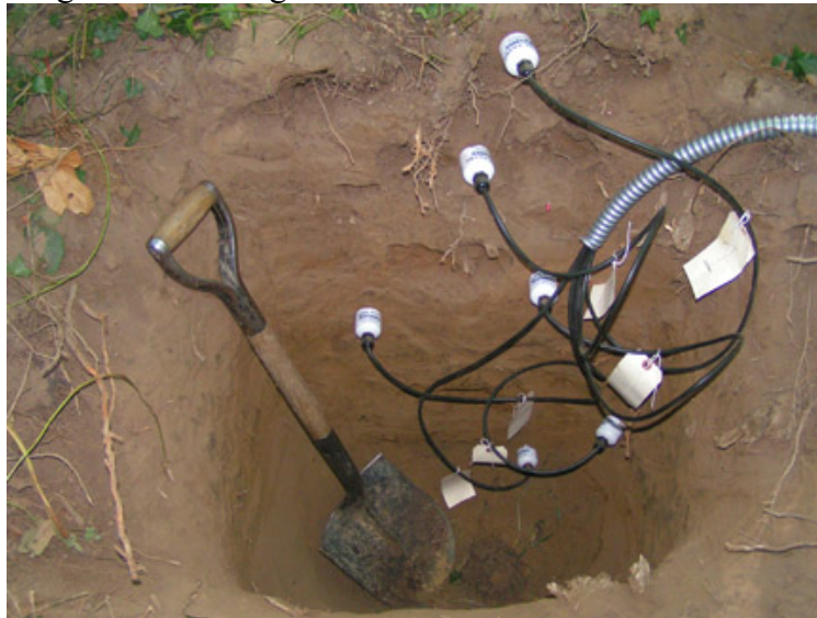
Figure 2.3 Six HydraProbes installed into 6 distinct soil horizons.
