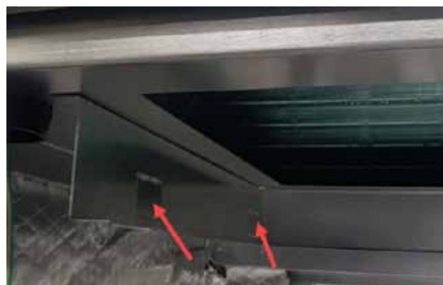
FIGURE 10 Bend Filter Tabs Down
