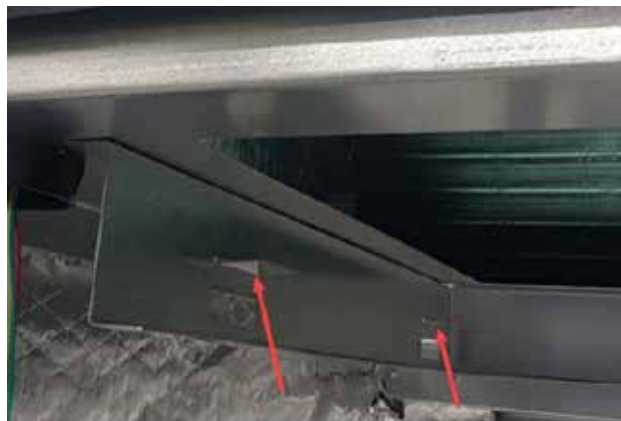
FIGURE 10 Bend Filter Tabs Down
