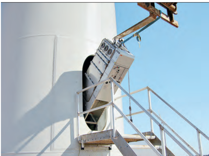
4 SafeWind, ABB's tailor-made switchgear for wind turbines, is the slimmest medium-voltage switchgear on the market.
