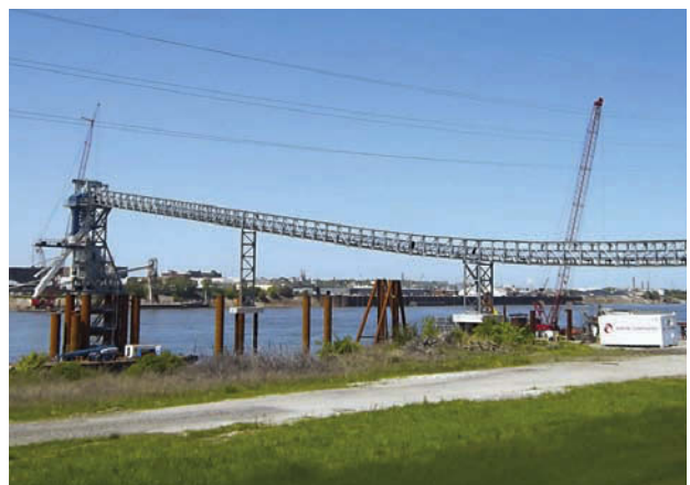
Barge load out conveyor system.
