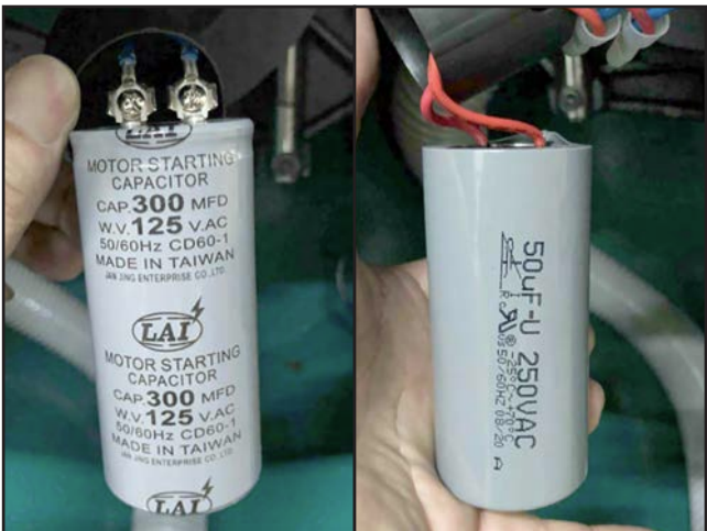
Figure 29. Start and run capacitors.
