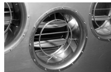
Figure 7. Flow-measuring OA damper
