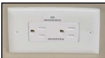
Figure 7-11. GFCI Receptacle
