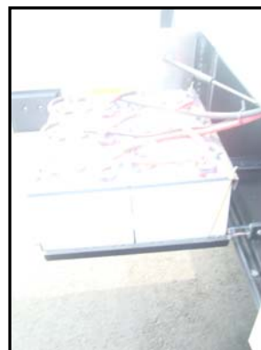
Figure 7-6. Batteries on Slide Tray
