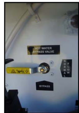
Figure 11-9. Water Heater Bypass System
