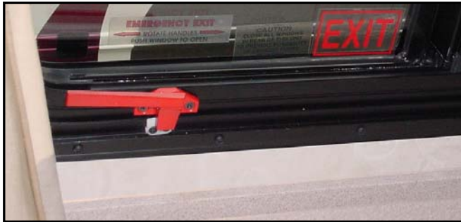
Figure 13-2. Bedroom Emergency Exit Window
