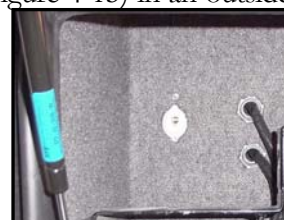
Figure 4-15. Cable & Telephone Jack
