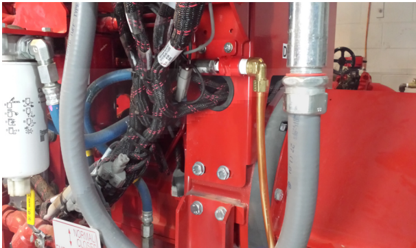
Figure 3-8 VSPLC Pressure Sensing Connection (optional)
