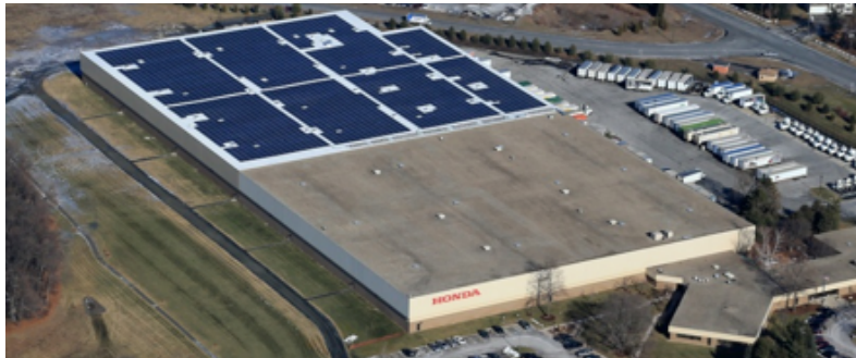
5,000 high-efficiency photovoltaic panels on Honda's Windsor Locks, Connecticut parts distribution facility.
