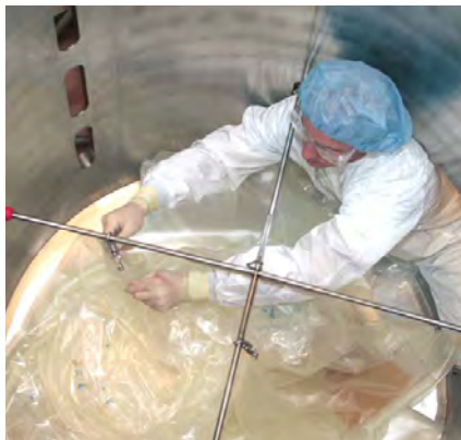
Figure 3.60. Connecting furthestmost retainer hooks.
