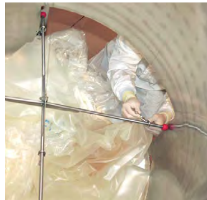
Figure 3.61. Connecting closest retainer hooks.
