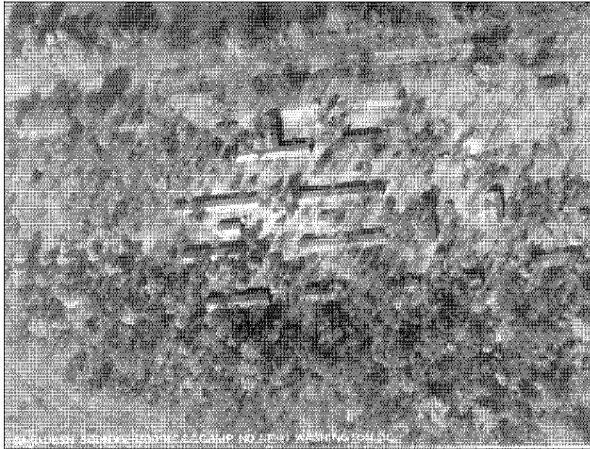
Figure 53: Camp NP-1-MD (C&O Canal), Aerial View, 1938. Source: RG 35-GE, Still Picture Branch, NARA.
