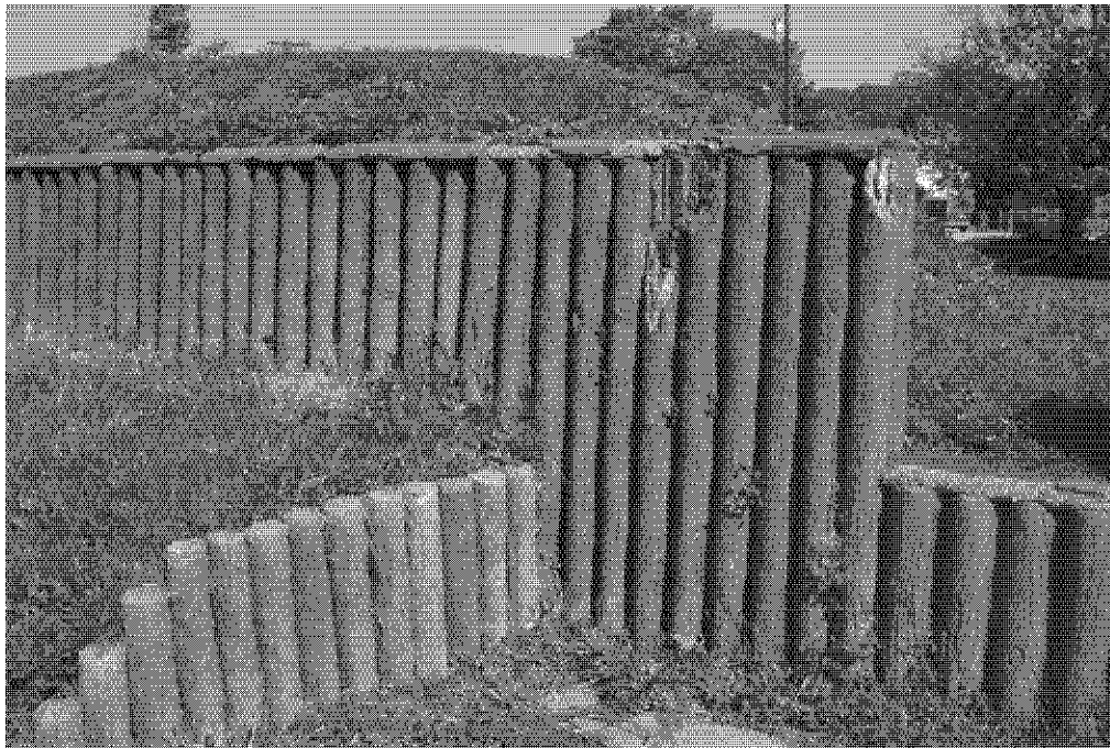
Figure 96: Ca. 1936 historical reconstruction of Fort Stevens using “concrete logs,” 2004.
