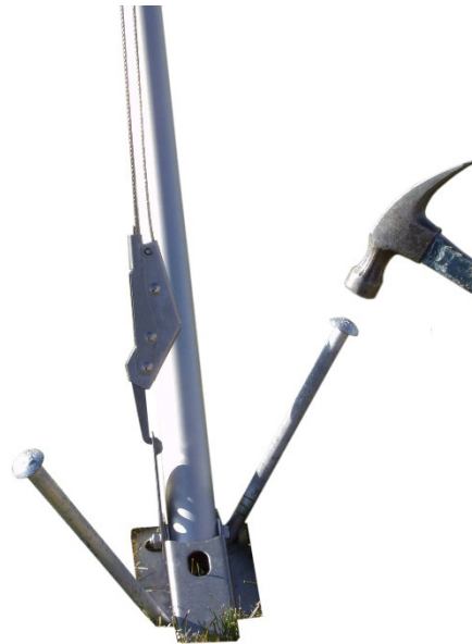
FIGURE 6-11. Staking the tripod feet
