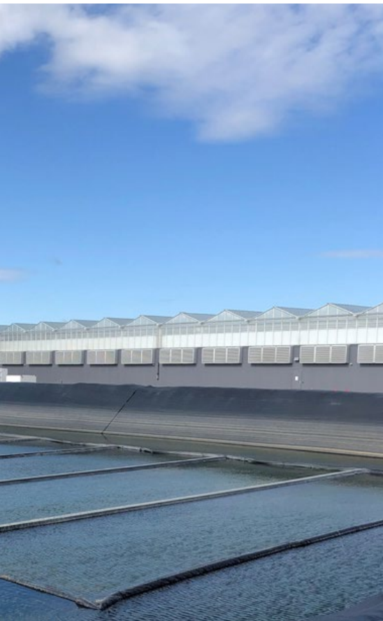
2. Rainwater reservoir currently in use at Aurora Sky.
