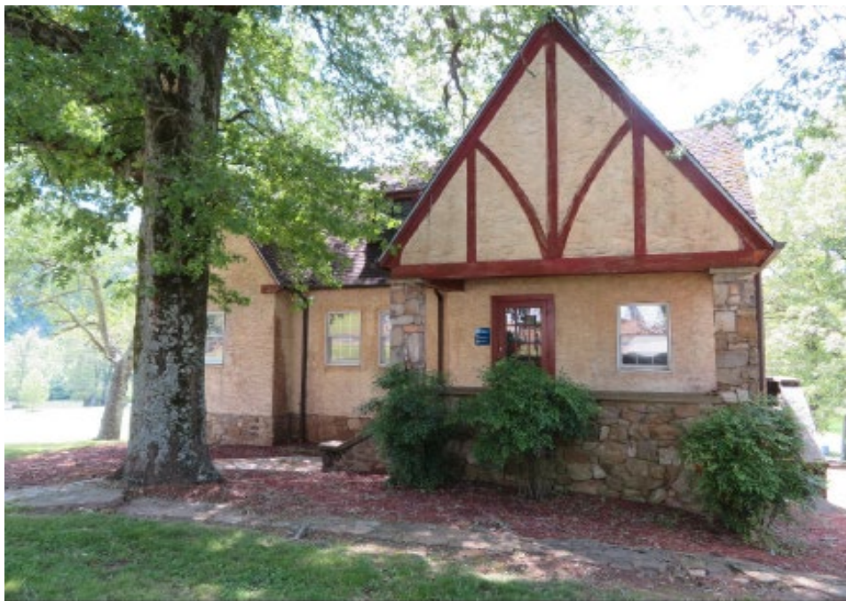
View of O1HTODA Building AEM8475 (Rock House/Ocoee Main Office), facing west/southwest.
