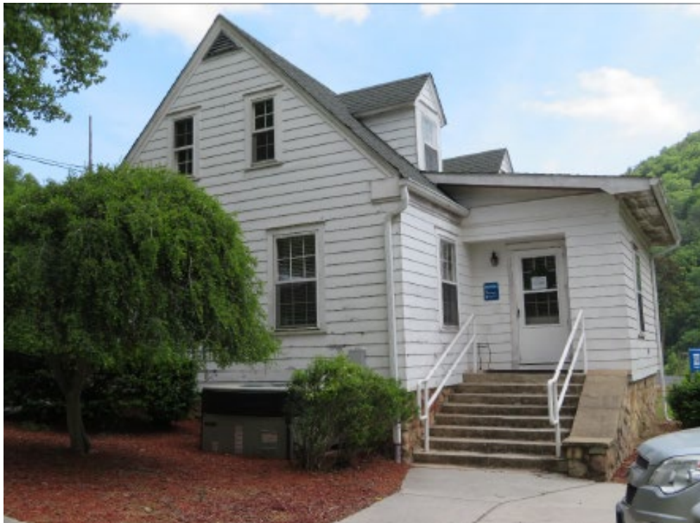
View of O1H Plant Office O1PO/Ocoee Regional Office, facing south/southeast.
