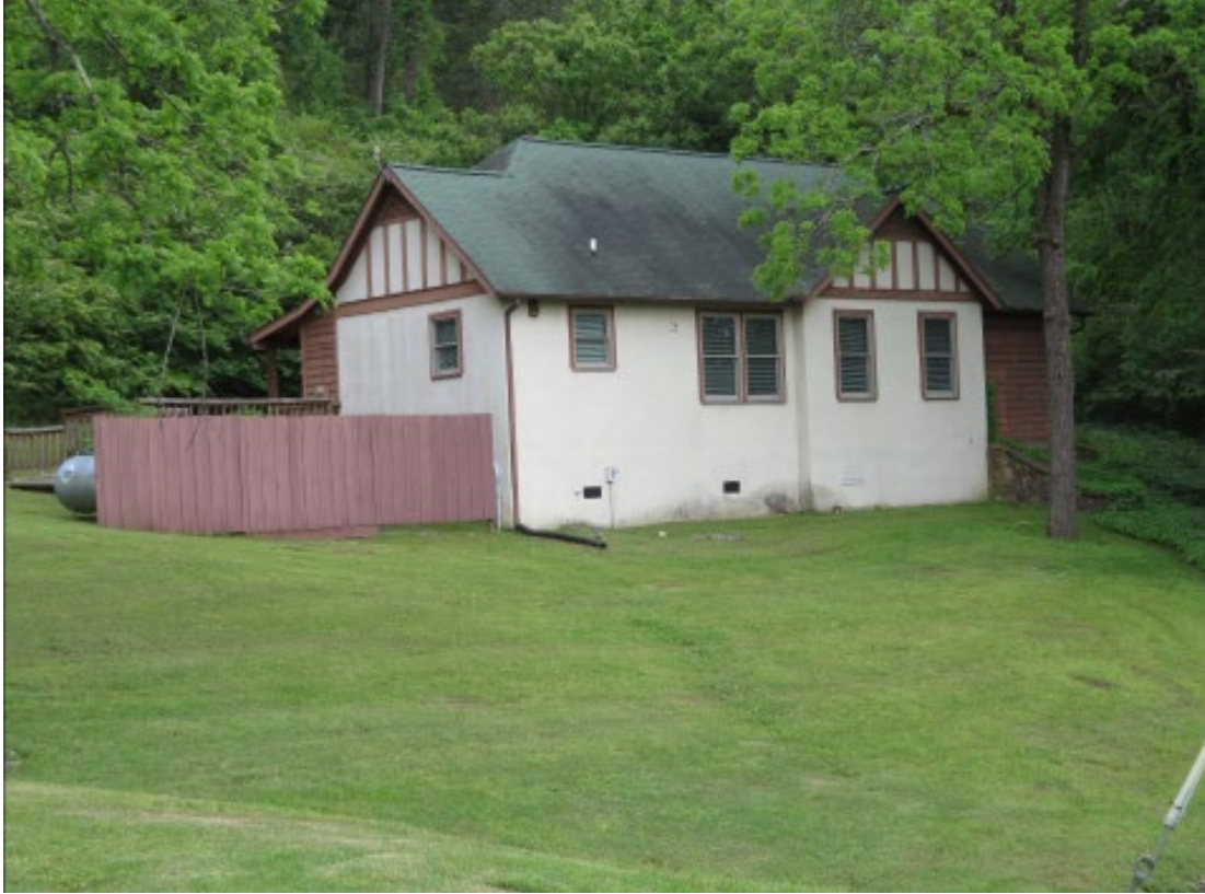
View of fourth house associated with O1H is located across the highway from the remainder of the O1H facility.
