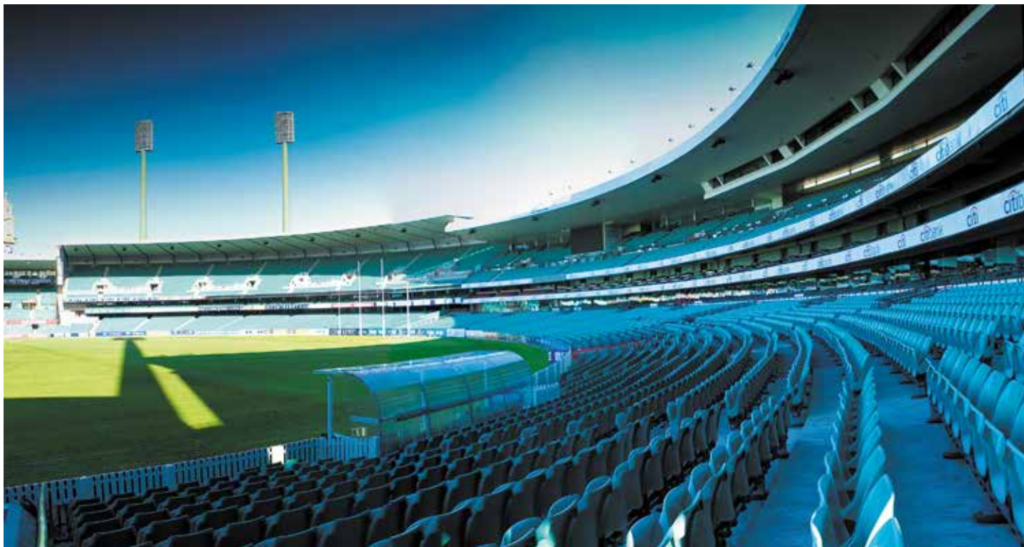
Sydney Cricket Ground features Zip Touch-Free washroom systems.
